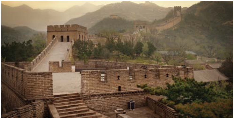
The Great Wall Of China
